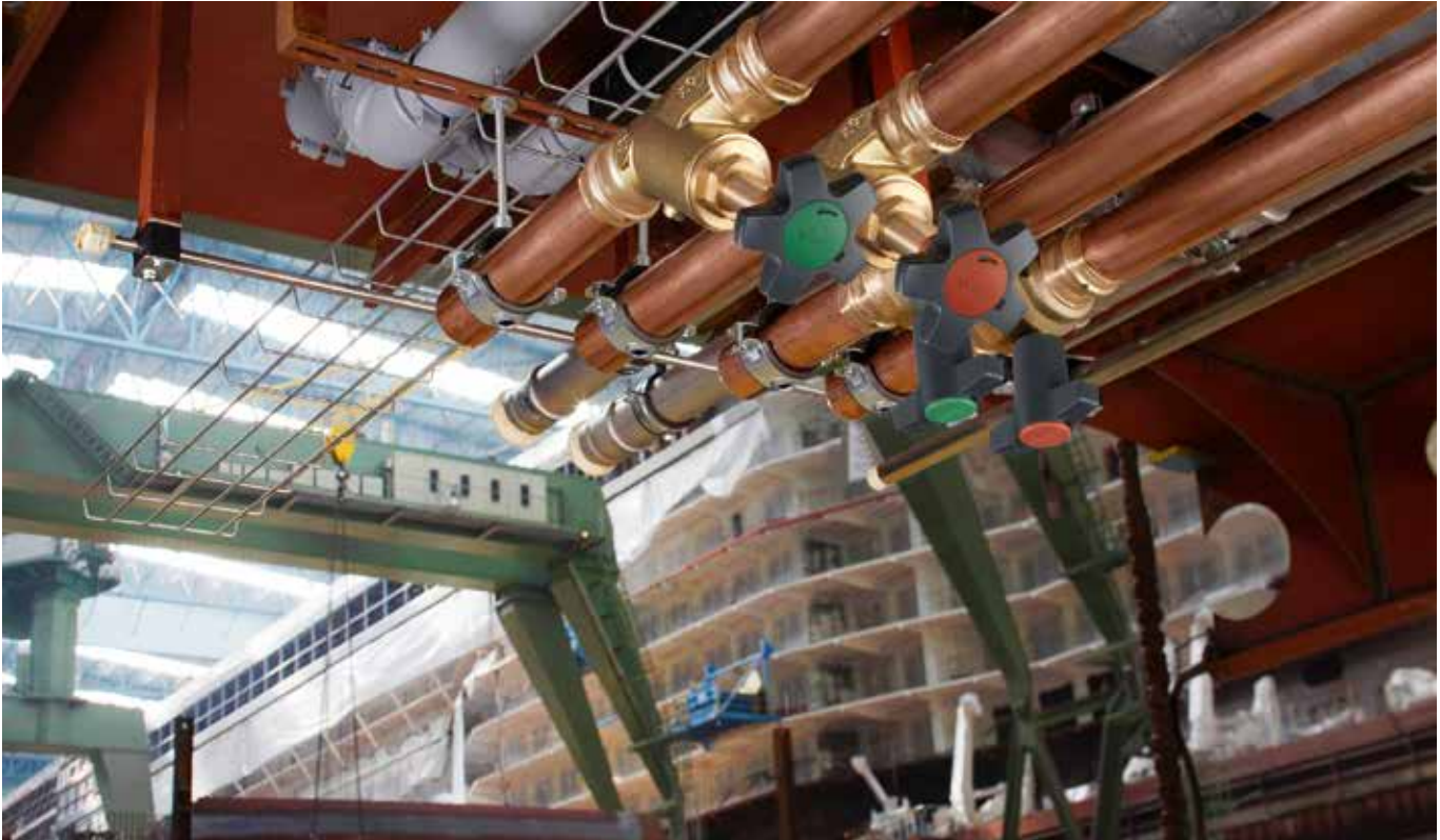
Supporting the construction of ocean-going cruise ships with Viega Profipress and Easytop at the Meyer shipyard, Papenburg.
